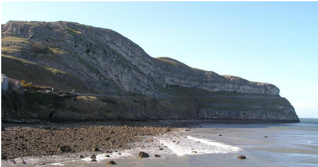
Cyclic stacking of Lower Carboniferous Limestone, Great Orme, Llandudno
